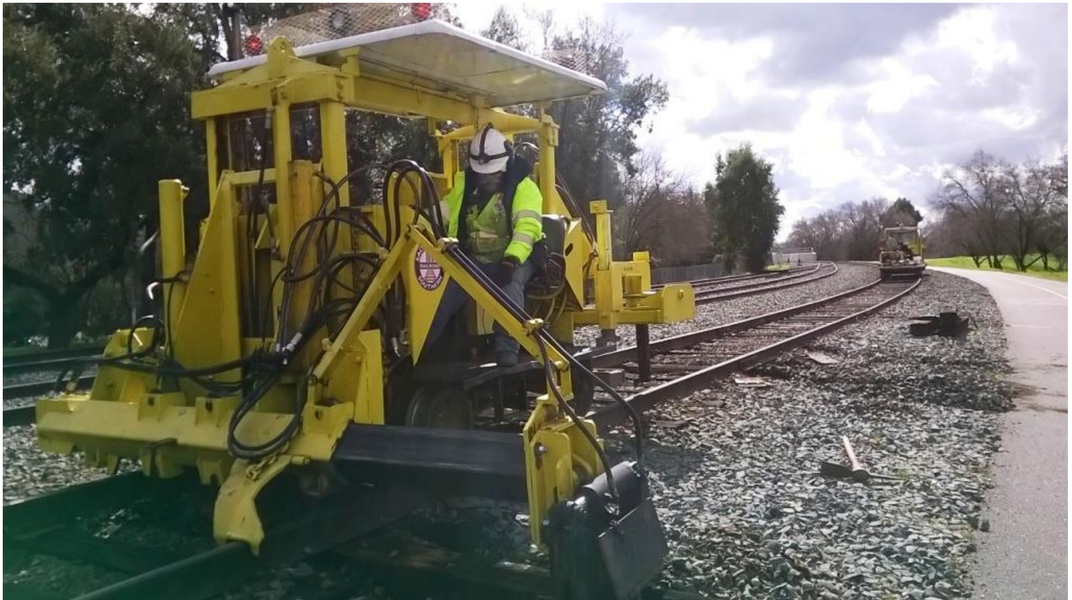
Joe, on the Jackson 125 tie-exchanger, pulls old rotten ties out from under the rails
