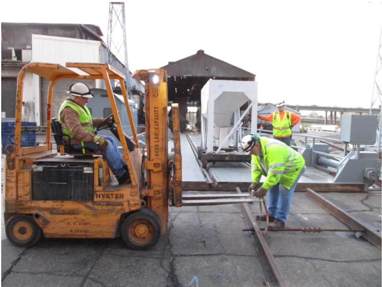
At the north end of the Erecting Shop, the temporary track needed to be relined so Frank hooks a strap to the forklift for Mike H. to move it
