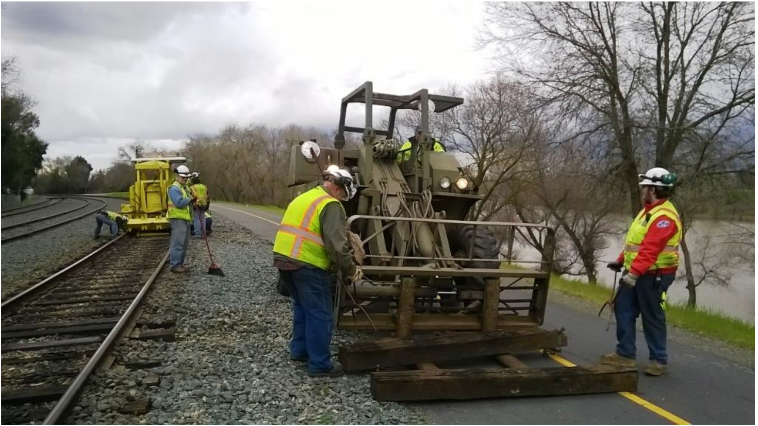
Art and Chris work with Mike F. on GM2 to load dead ties for disposal
