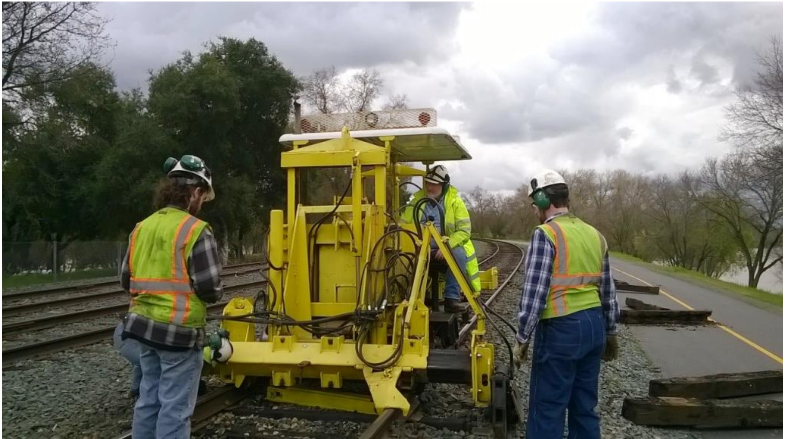
Matt and Weston work with Frank to insert tie-plates as the Jackson 125 lifts the rails with its jacking system
