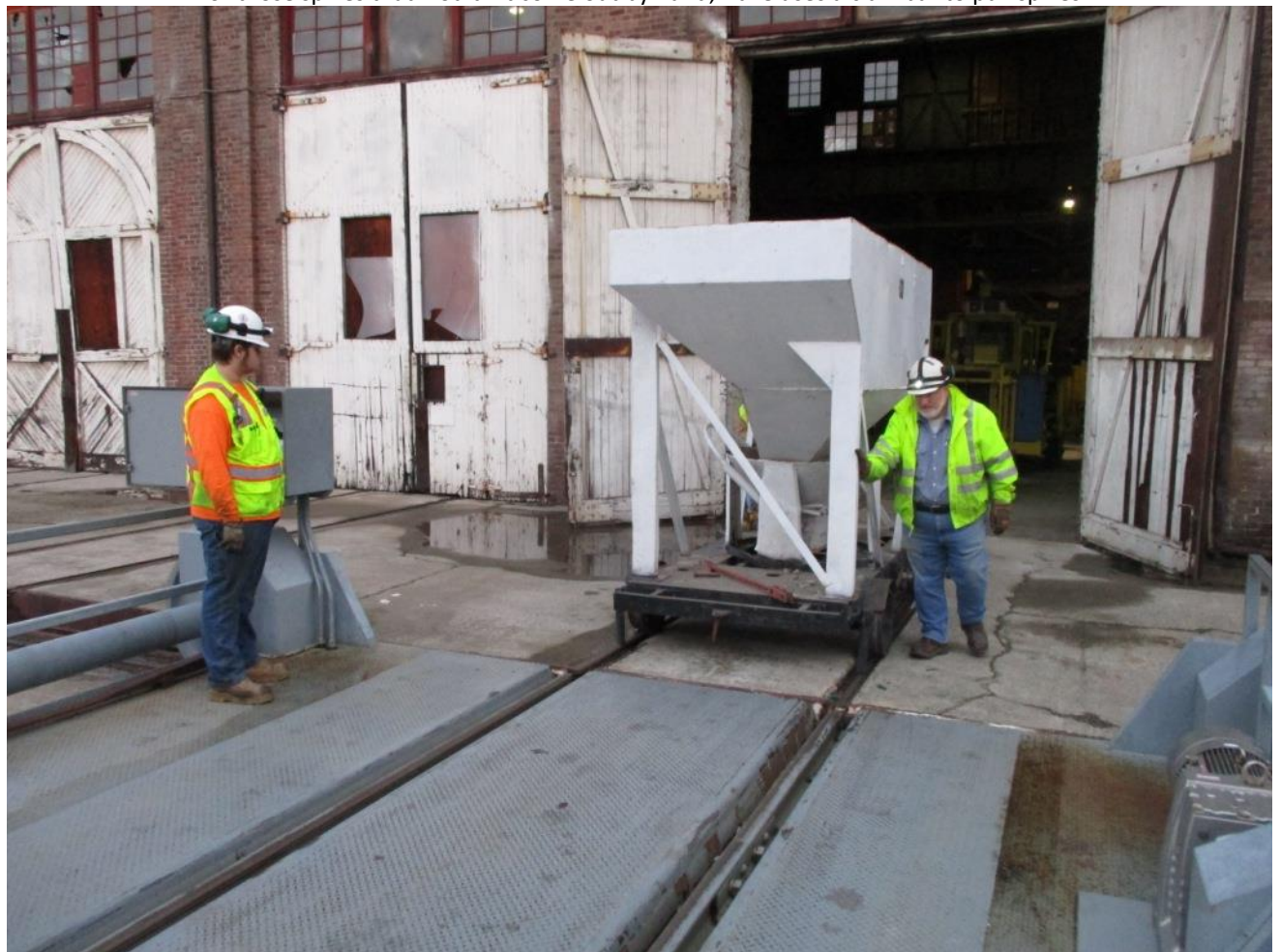
Chris H. brings in the transfer table as Frank pushes the ballast hopper car out of the Erecting Shop
