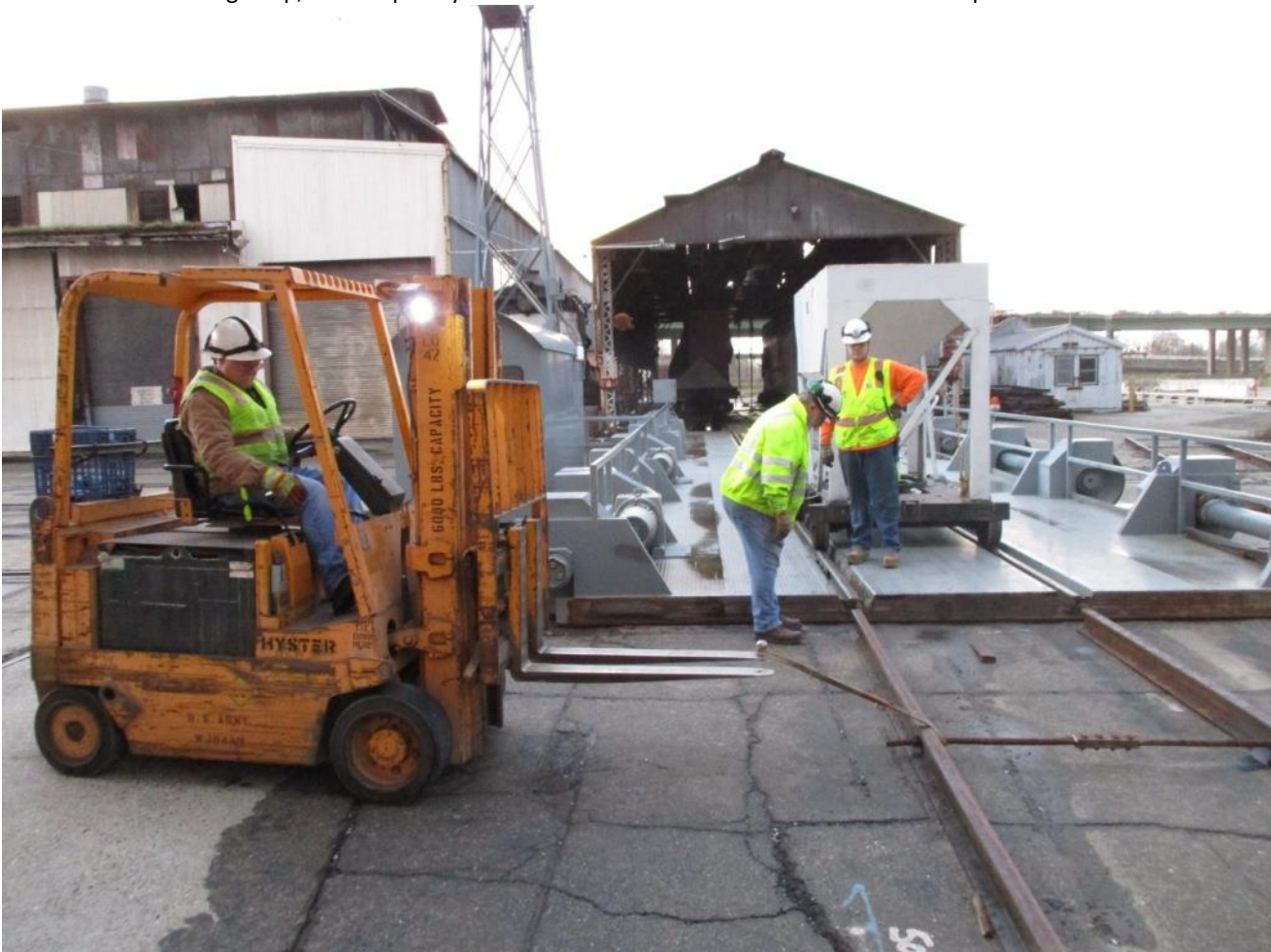
Frank verifies that the rails line up as Mike H. moves the track with the forklift
