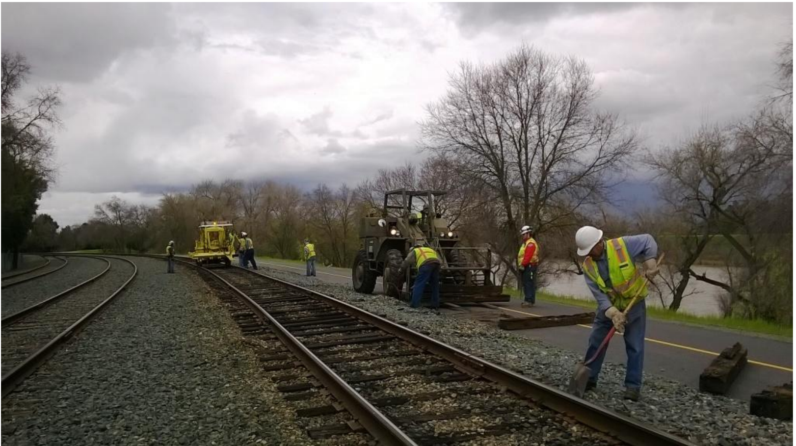
Your MOW Team at work: Joe, Frank, Matt, Weston, and Mike W. plate ties; Mike F., Art and Chris H. load dead ties; Mike T. fills in holes
