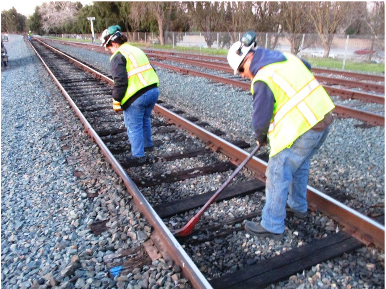
For those spikes that wouldn't come out by hand, Dave uses a claw bar to pull spikes
