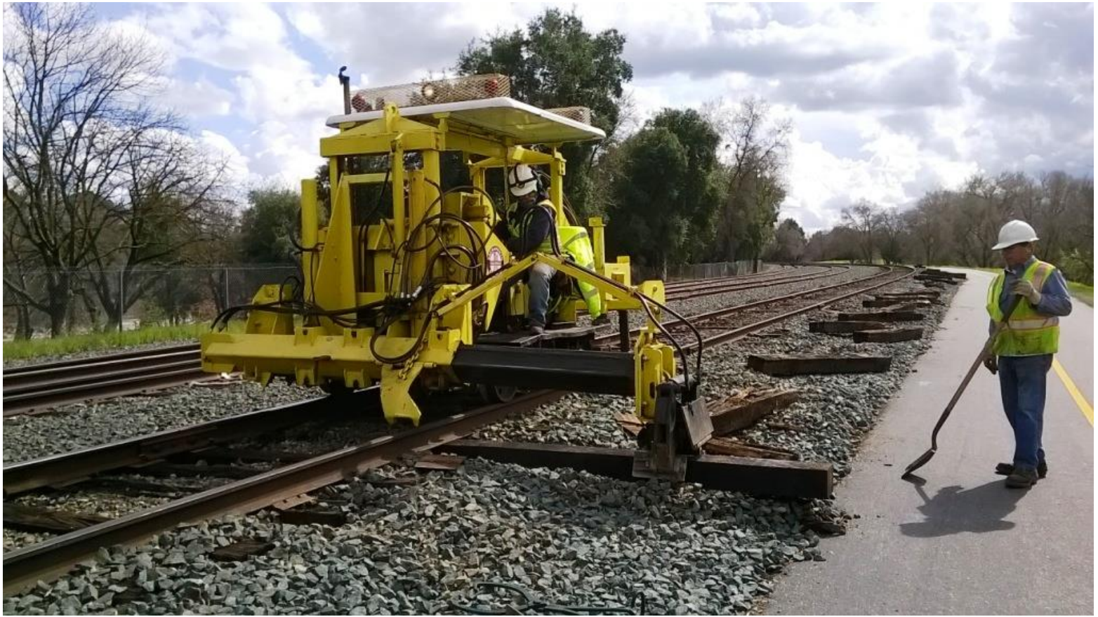
...Which Joe pulls into place
